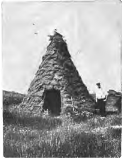
FIG. 18.—The oldest house, that of the charcoal-burner (England); it is a teepee tent in stone.
